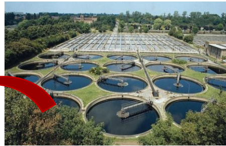
Wastewater Treatment Plant (WWTP)
